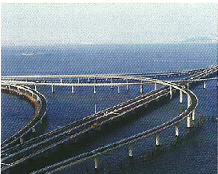
照明产品应用于青岛胶州湾跨海大桥 Lighting Fixture Products Are Applied to Jiaozhou Cross-sea Bridge, Qingdao
