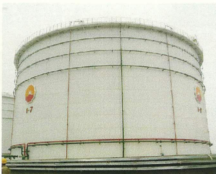
战略油库光纤温度监测 Optical Fiber Temperature Monitoring for Strategic Oil Depots
